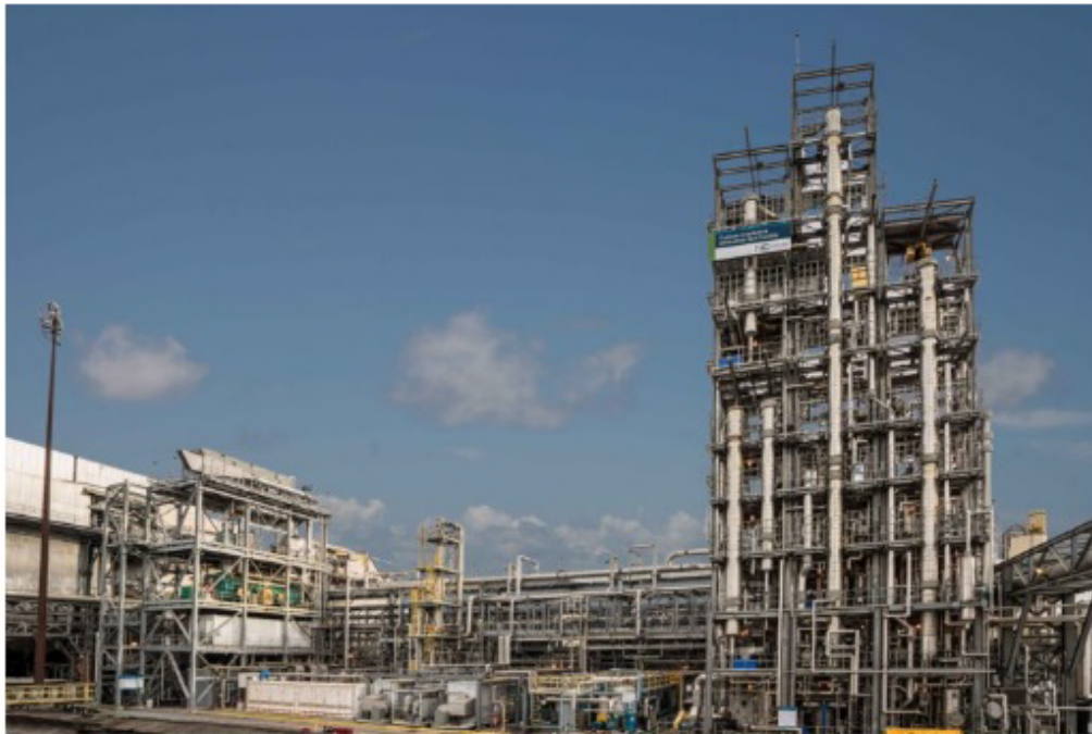
National Carbon Capture Center test facility, Wilsonville, Alabama
