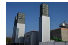
Combustion Test Center in Berlin
